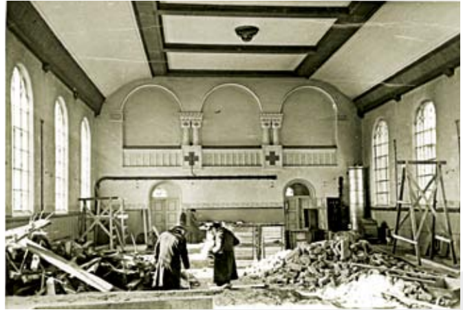
Remodeling the sanctuary into a TV studio - 1961
