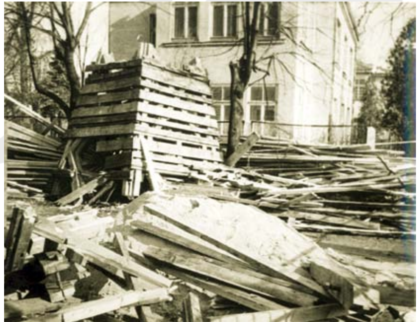
Removing the steeple -1965
