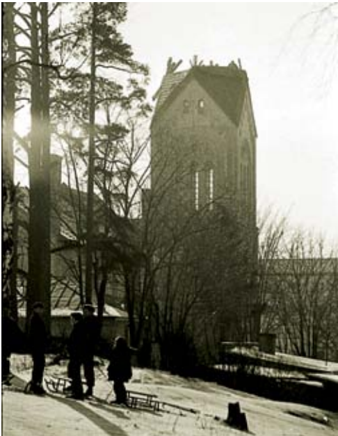
Removing the steeple -1965
